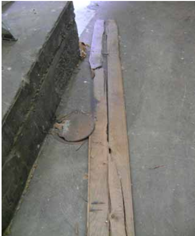
Photo 17 - Located near the roller door, access off Fred Street
