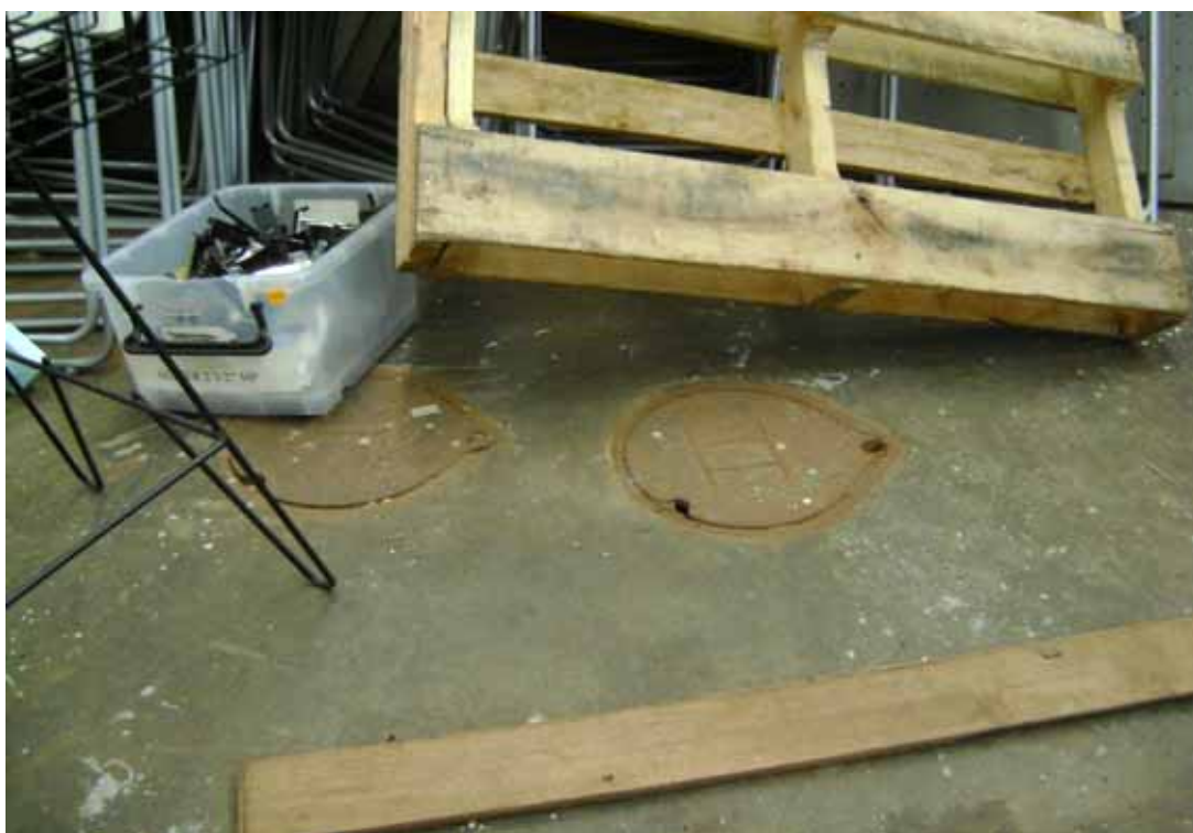
Photo 16 - Dip and fill points were identified near the roller door entrance from Fred Street
