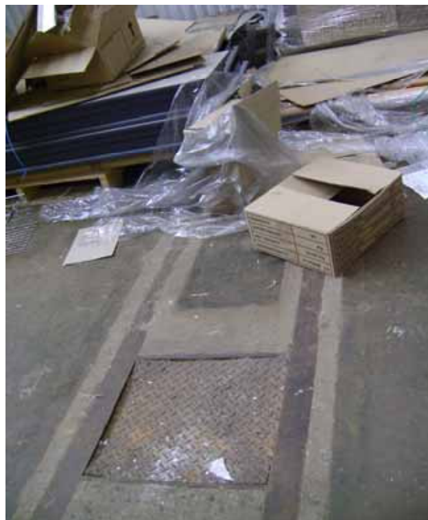
Photo 18 - North eastern portion of warehouse
