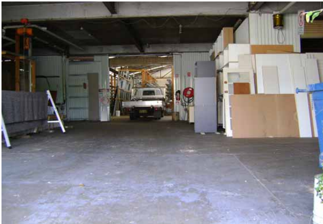
Photo 4 - looking into warehouse from Alberto Street
