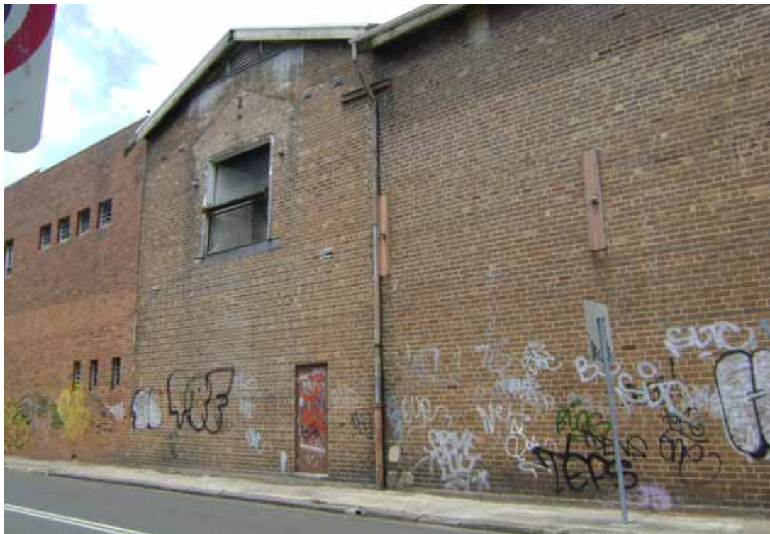
Photo 12: Cecily St frontage. Remains of delivery hoist area evident
