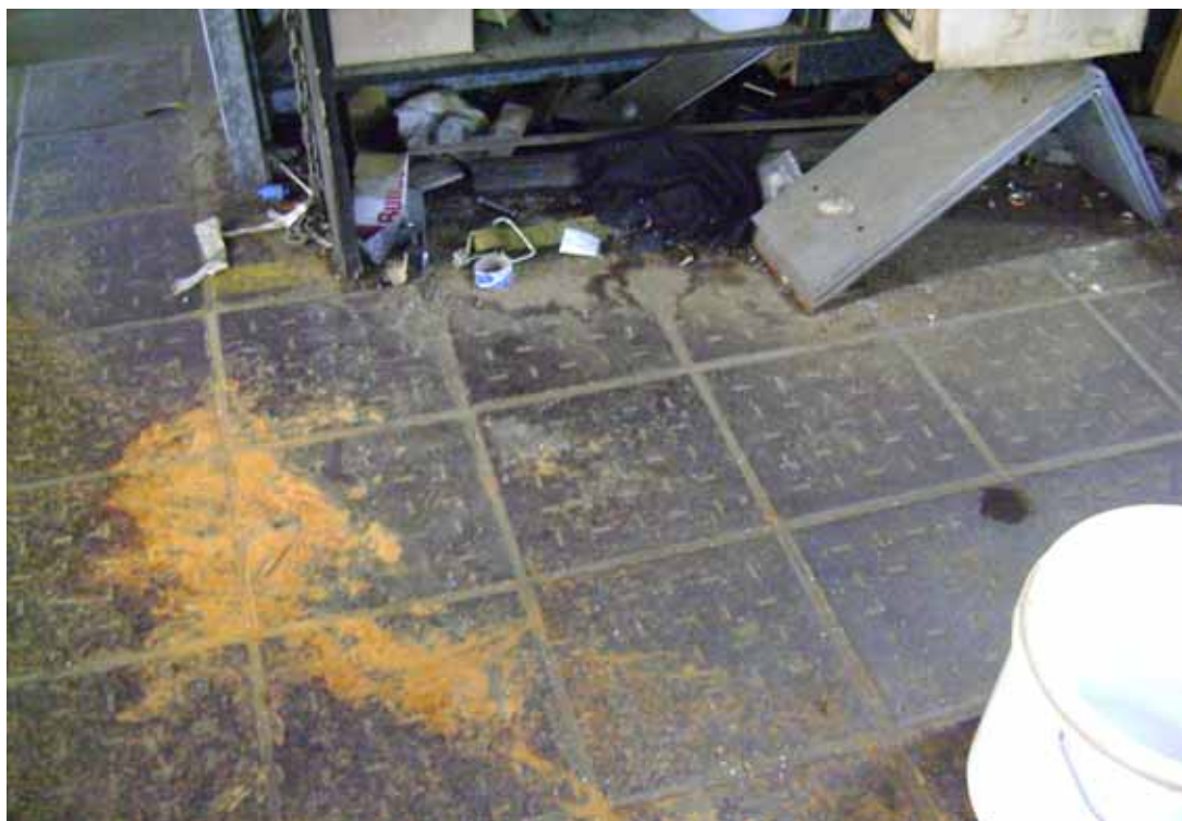
Photo 5 - steel flooring and staining in warehouse off Alberto St
